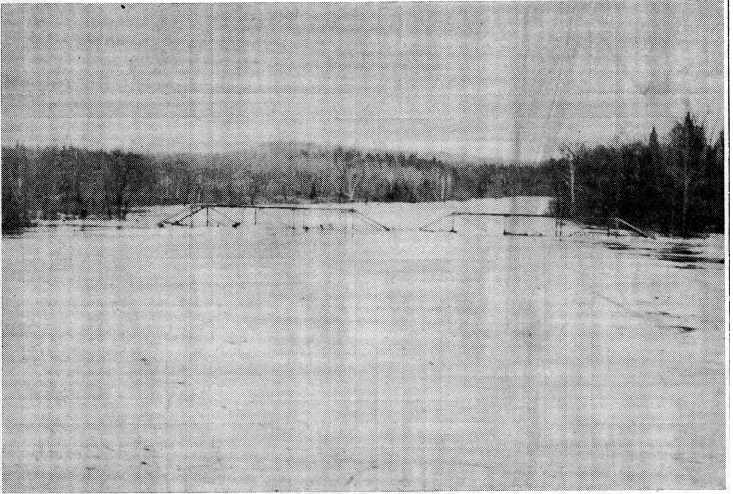
NO CLEARANCE —The normal clearance between the Bates-Amasa bridge on county road 643 and the Paint river which it spans is 11 feet. When this picture was taken a week ago Monday, water was up to the hand rails.
