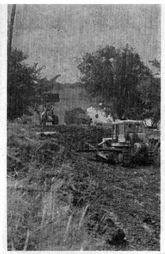
ROAD REBUILDING PROJECT — Crystal Falls township contracted with the Road Commission recently for the complete reconstruction of a troublesome stretch of the Ski Hill Road north of Forest Avenue, and tons and tons of unstable ground had to be dug out before an adequate base
