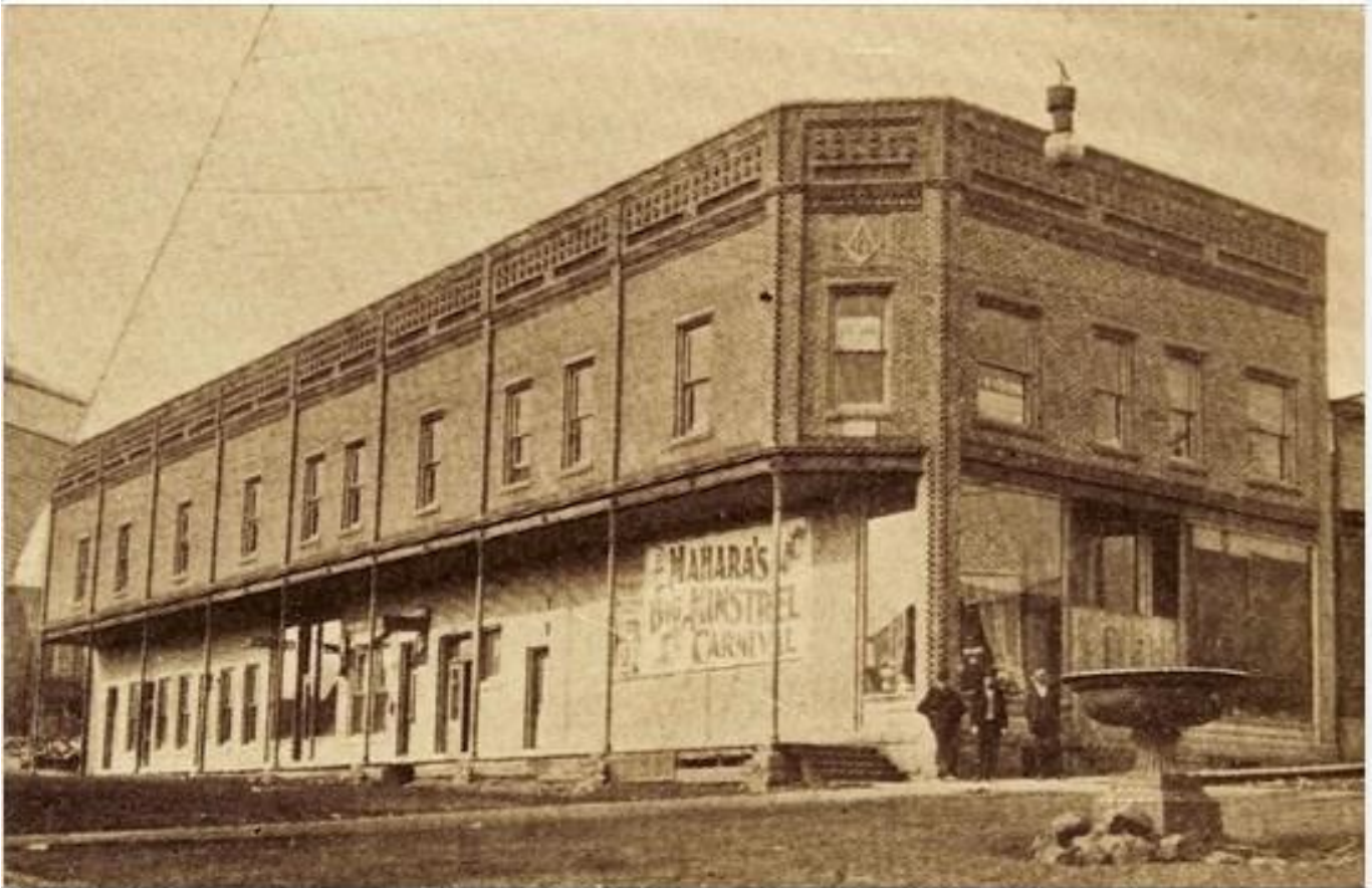
This building is where the Ben Franklin store is now in Crystal Falls
